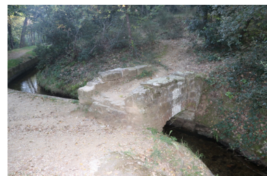
Canal de Bohère - Ponceau 6 (a). Phot. Léonie Deshayes IVR76_20216661943NUCA
