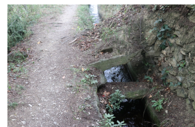
Canal de Canoha - Ponceau 2. Phot. Léonie Deshayes IVR76_20216661955NUCA
