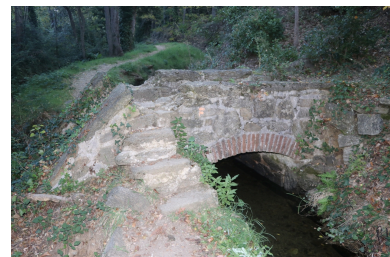
Canal de Bohère - Ponceau 4 (a). Phot. Léonie Deshayes IVR76_20216661940NUCA
