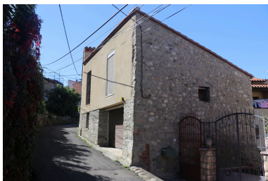
Moulin à farine communal - Façade Est. Phot. Léonie Deshayes IVR76_20216665025NUCA
