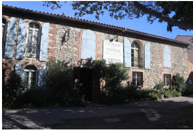
Tannerie Guitard - Façade Ouest. Phot. Léonie Deshayes IVR76_20216665097NUCA
