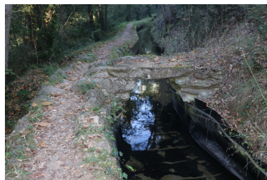
Canal de Bohère - Ponceau 3. Phot. Léonie Deshayes IVR76_20216661939NUCA
