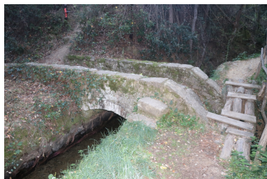
Canal de Bohère - Ponceau 2. Phot. Léonie Deshayes IVR76_20216661938NUCA
