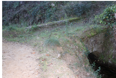
Canal de Bohère - Ponceau 1 (a). Phot. Léonie Deshayes IVR76_20216661936NUCA
