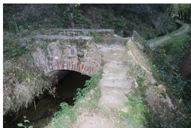
Canal de Bohère - Ponceau 4 (b). Phot. Léonie Deshayes IVR76_20216661941NUCA
