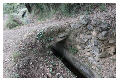
Canal de Canoha - Ponceau 1. Phot. Léonie Deshayes IVR76_20216661954NUCA
