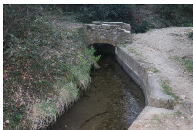
Canal de Bohère - Ponceau 6 (b). Phot. Léonie Deshayes IVR76_20216661944NUCA
