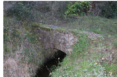
Canal de Bohère - Ponceau 1 (b). Phot. Léonie Deshayes IVR76_20216661937NUCA
